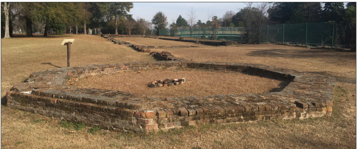
C. View of Arsenal Compound Wall and Southwest Tower Looking Northeast
